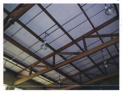
TECTUM Inc. has been in business since 1949 offering a cementitious wood fiber acoustical Roof Deck as an alternative to Steel Deck. With the unpredictable price of BA deck or other acoustical steel decks, and the short supply of steel, Tectum Roof Deck is your answer. New ANSI S2.60.2002 guidlines that address acoustical performance in schools can be easily and effectively addressed using a Tectum Roof Deck. Tectum Roof Deck products are considered "green" and contribute to the LEED program.
